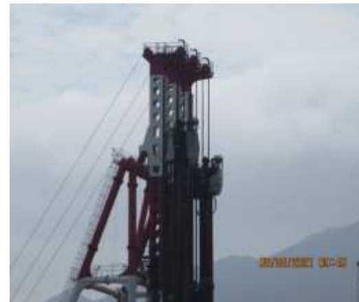
Noise mitigation measures on deep cement mixing plant
