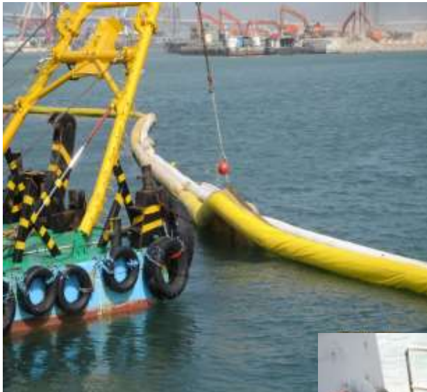
Maintenance of perimeter silt curtain
