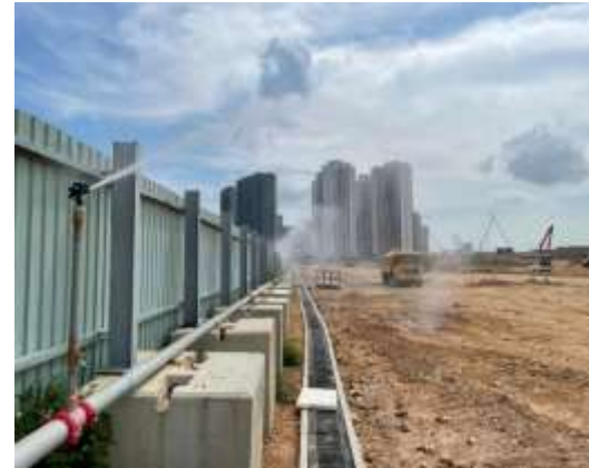
Automatic sprinklers for dust control
