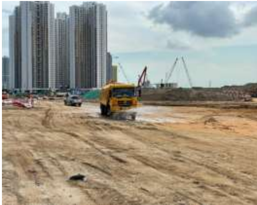
Water spraying by water truck for dust control
